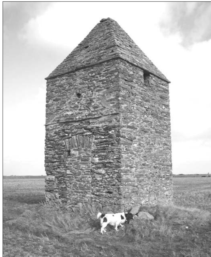
Signal Station at West Soar showing evidence of a previous adjoining building and high window through which a telescope protruded.
