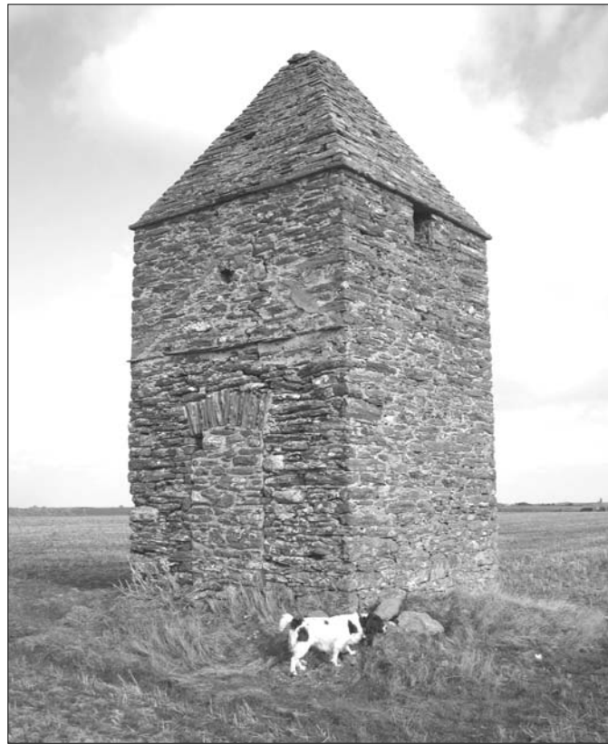
Signal Station at West Soar showing evidence of a previous adjoining building and high window through which a telescope protruded.
